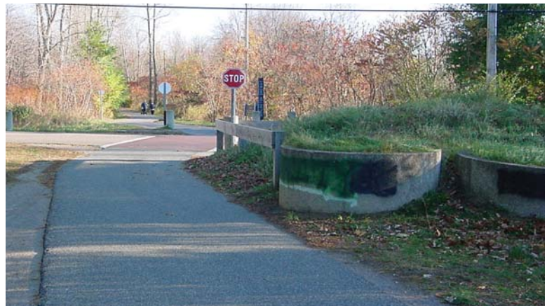
Figure 12: Poor Sight Distance at Staniford Road Intersection
