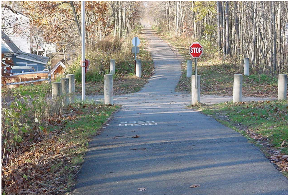
Figure 13: Looking North at the North Ave. Extension Intersection
